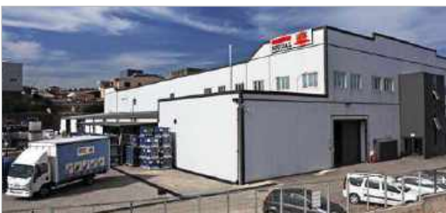
Soudal sealant production: Istanbul (Turkey)
