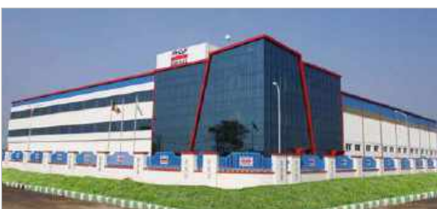
McCoy Soudal Plant and R&D Centre (Bawal), Haryana
