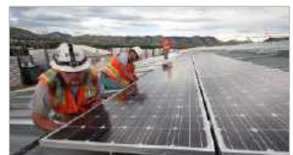
Frame to module bonding & sealing
