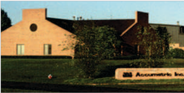
Soudal sealant production: Elizabethtown (USA)
